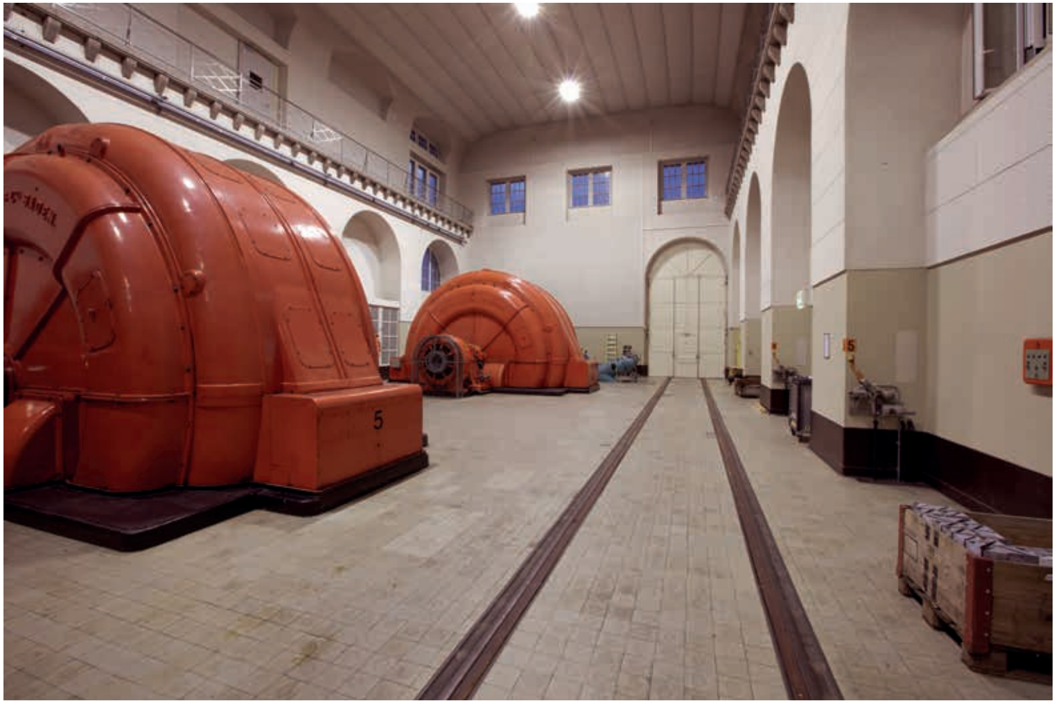
Pictures: Ritom hydroelectric plant, above Piotta
